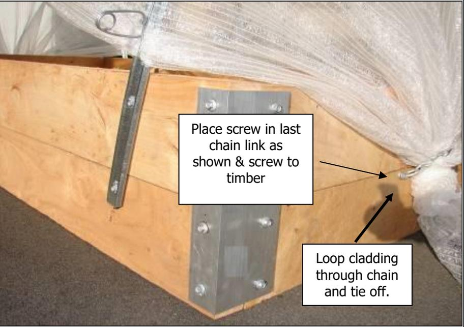
Place screw in last chain link as shown & screw to timber
