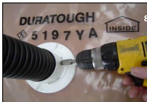
Position a Tek screw to secure all of the parts together in case of high wind load
