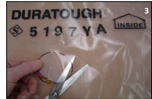
Cut out the 60mm hole, taking care not to accidentally cut the outer twinskin cover.
