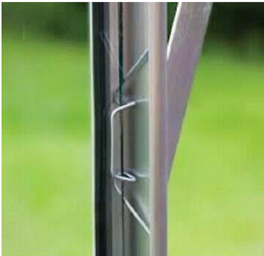
Images of wire butterfly clips to hold cladding:
