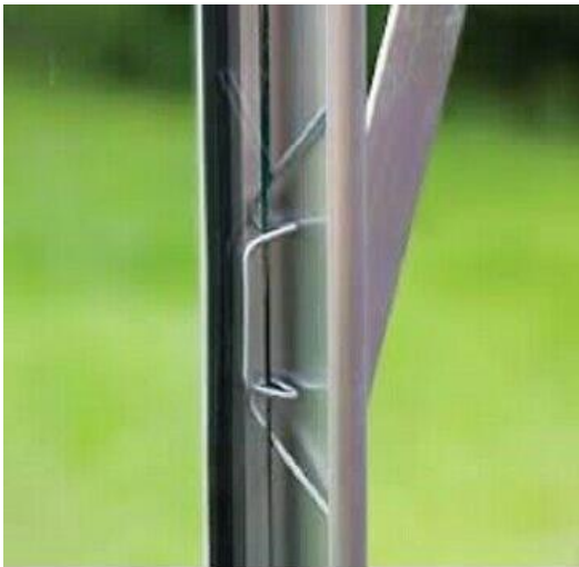
Images of wire butterfly clips to hold cladding:
