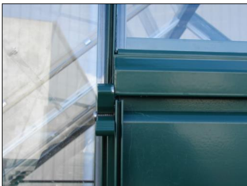
Align end of door track with door in fully closed position.
