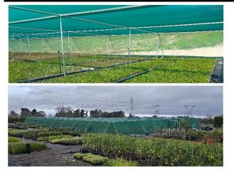
Our popular Quickbuild Shadehouse are a costeffective and a simple to build "sleeve-connected" all steel frame design.
