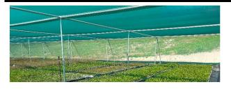
Used to shelter from the sun, Dairy herds, Beef, Goats etc, We supply them in a range of modular sizes to suit the individual needs. Our design includes simple slide-together connectors for quick and secure assembly of the main frame. Only basic tools and skills are needed to erect the building. The Redpath Shadehouses give owners speedier build times, improved durability and affordability over more traditional timber pole/wire & clip designs.
