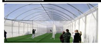
Redpaths specialist Duratough heavy duty long life clear roof cladding allows PAR (photosynthetic active radiation) light to travel through the cladding which in-turn allows natural grass pitches to be grown within the shelter if required. Artificial turf is also a common use within the Redpath cricket shelters. Natural light provides life-like conditions for bowlers and batsmen to practice.
