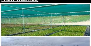
Our popular Quickbuild Shadehouse are a costeffective and a simple to build "sleeve-connected" all steel frame design.
