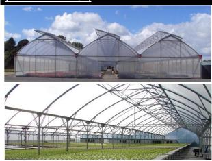
Top of the line greenhouse models from Redpath. They are fully NZ building code compliant design engineered structures, utilising strong RHS steel, HDG poles, 12mm fully bolted 4mm plate connections, and cold rolled 'walk-through' wide steel gutters as standard.
